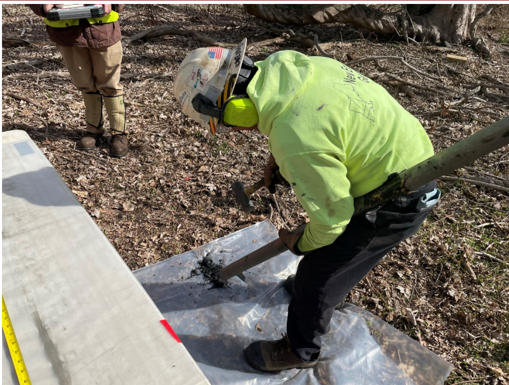
2. View of New England Geotech extruding contents of last core for 11SB1
