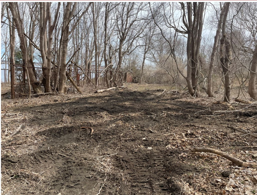
4. View of cleared path to NED 13
