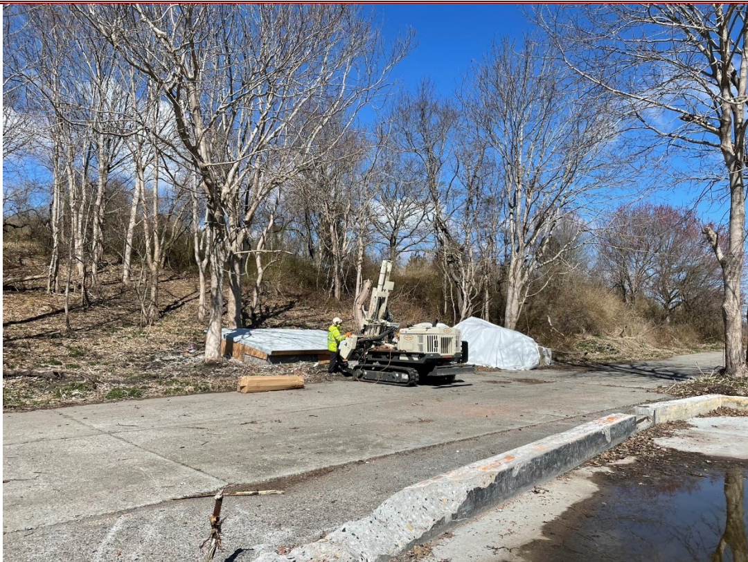
4. View of angled boring advancement at the Switch House (NED 50)
