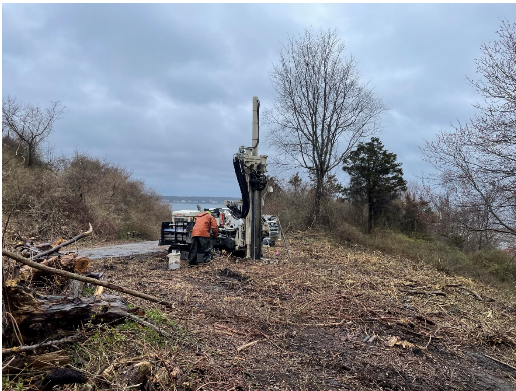
1. View of boring advancement at NED 01
