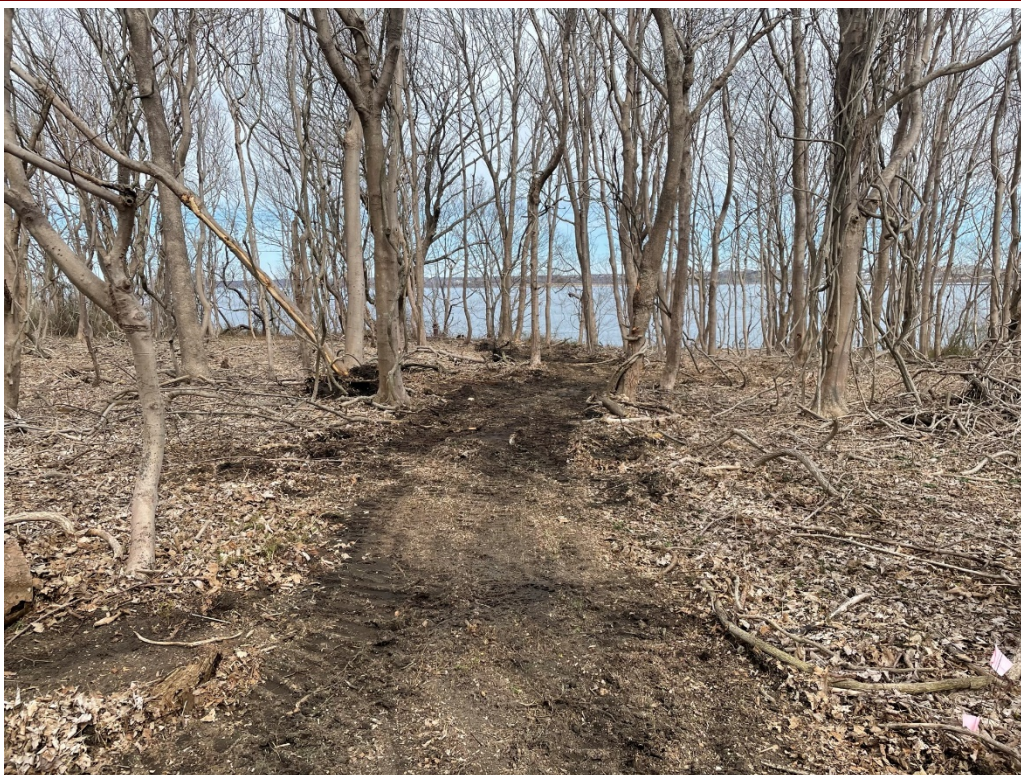
2. View of cleared path to 11OBMW1 location
