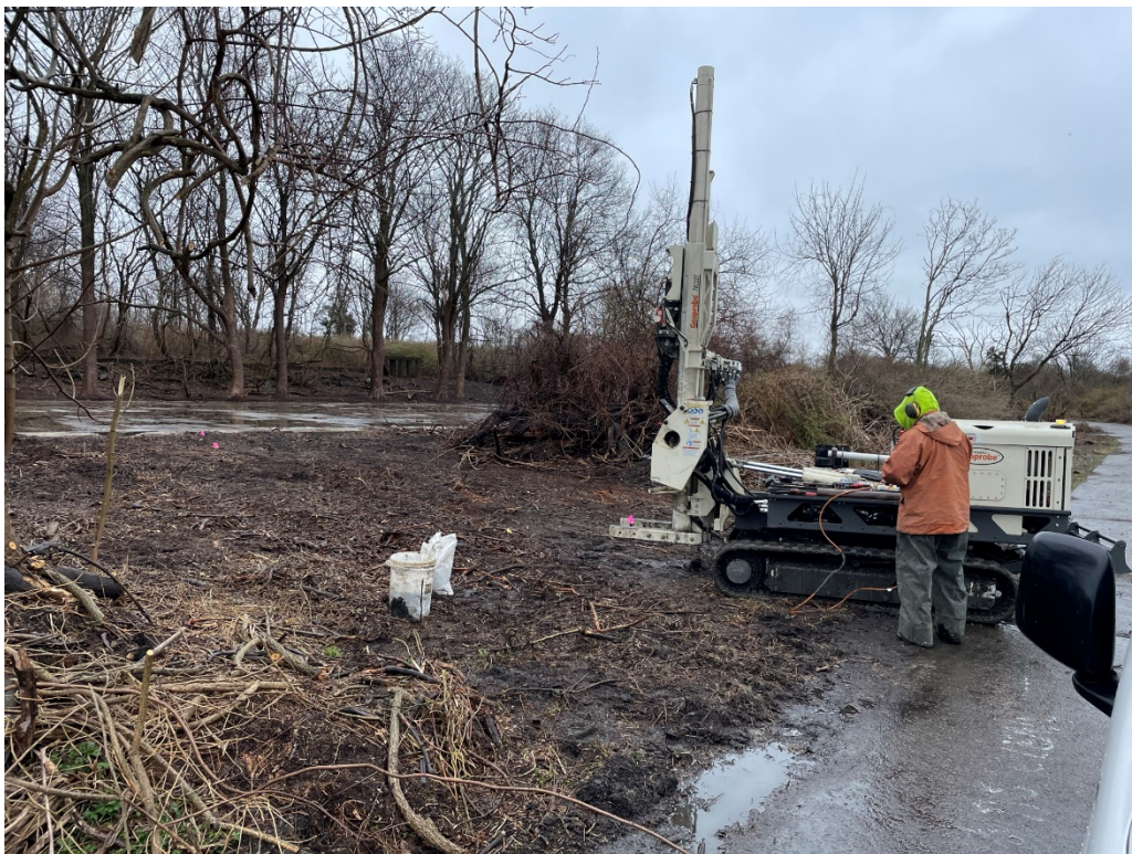
3. View of boring advancement at NED 38
