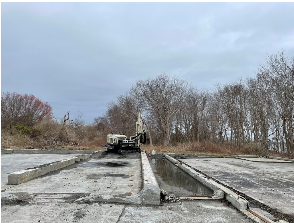
1. View of boring advancement at NED 12
