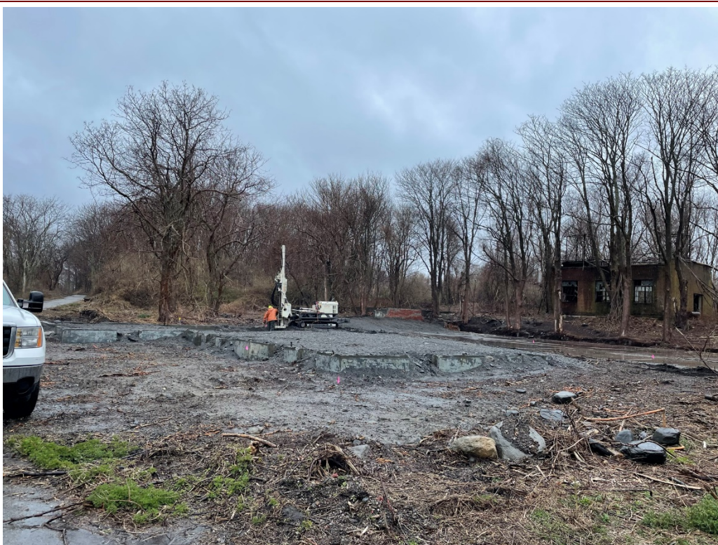
2. View of boring advancement at NED 36
