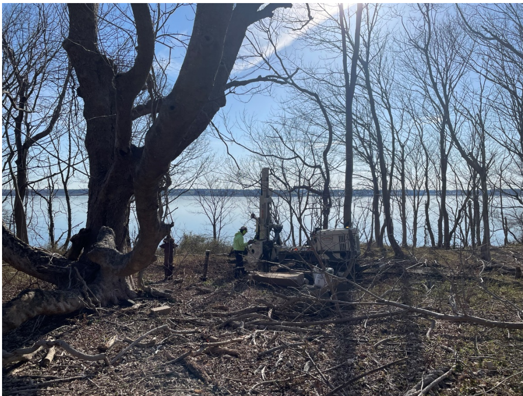
1. View of boring advancement at 11SB1
