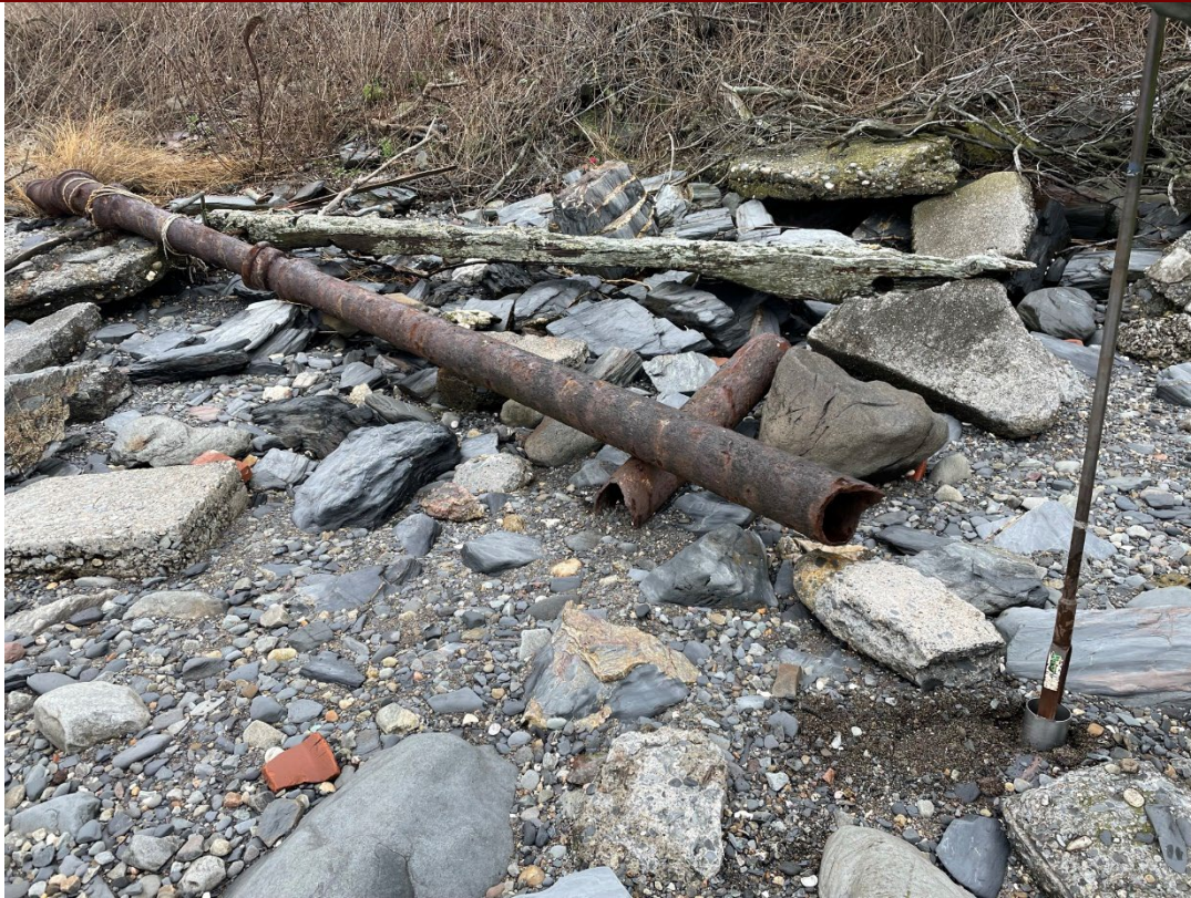
11. View of outfall sampling at non-submerged location (OF-10)
