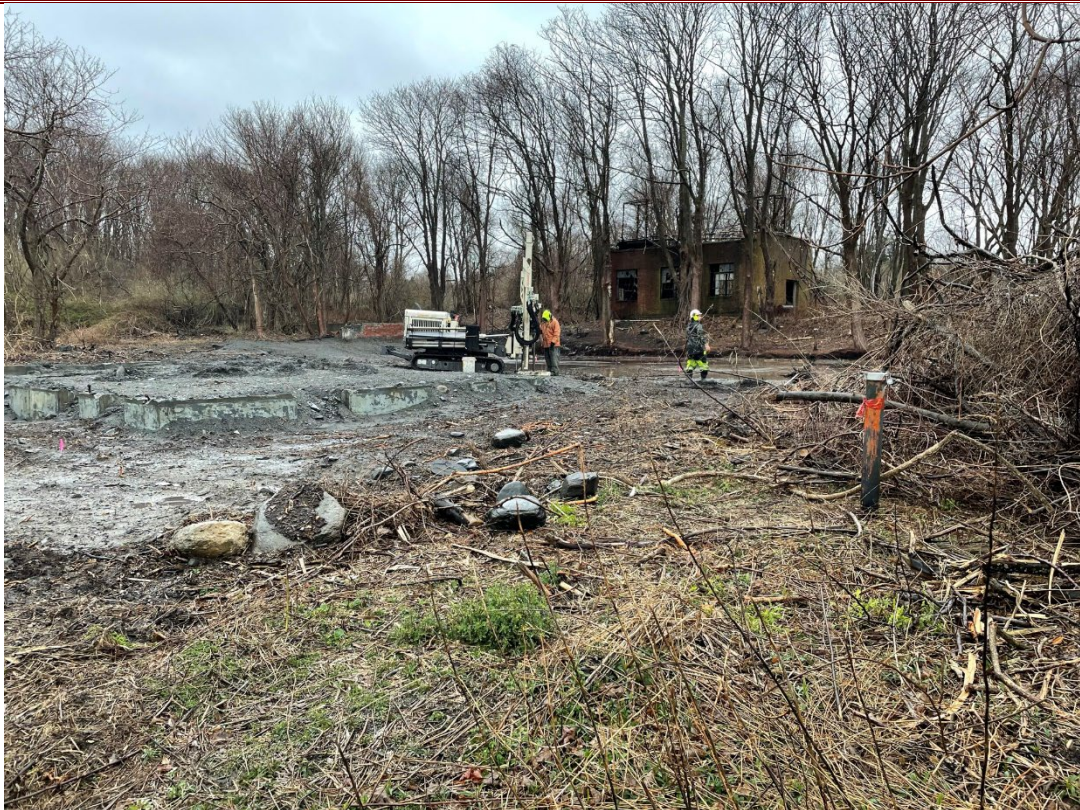
8. View of boring advancement at Degaussing Building/Torpedo Building (NED 36/38)
