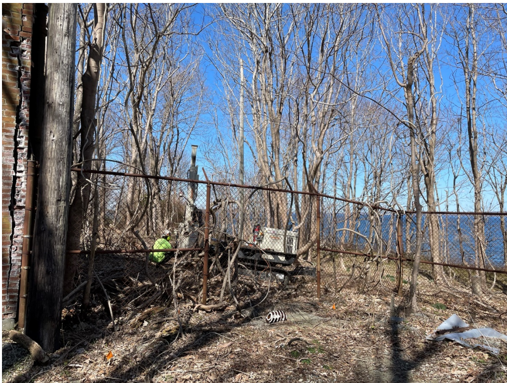
3. View of boring advancement at NED 13
