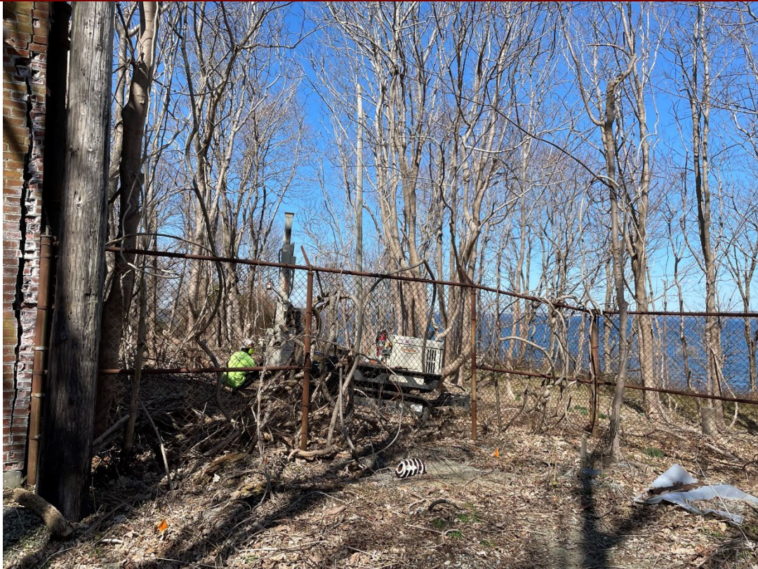
5. View of boring advancement at Transformer Pen (NED 13)
