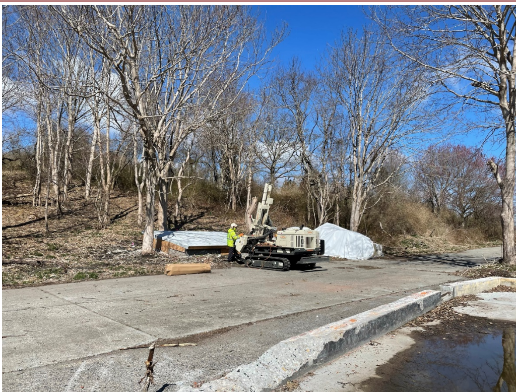
2. View of angled borings at NED 50
