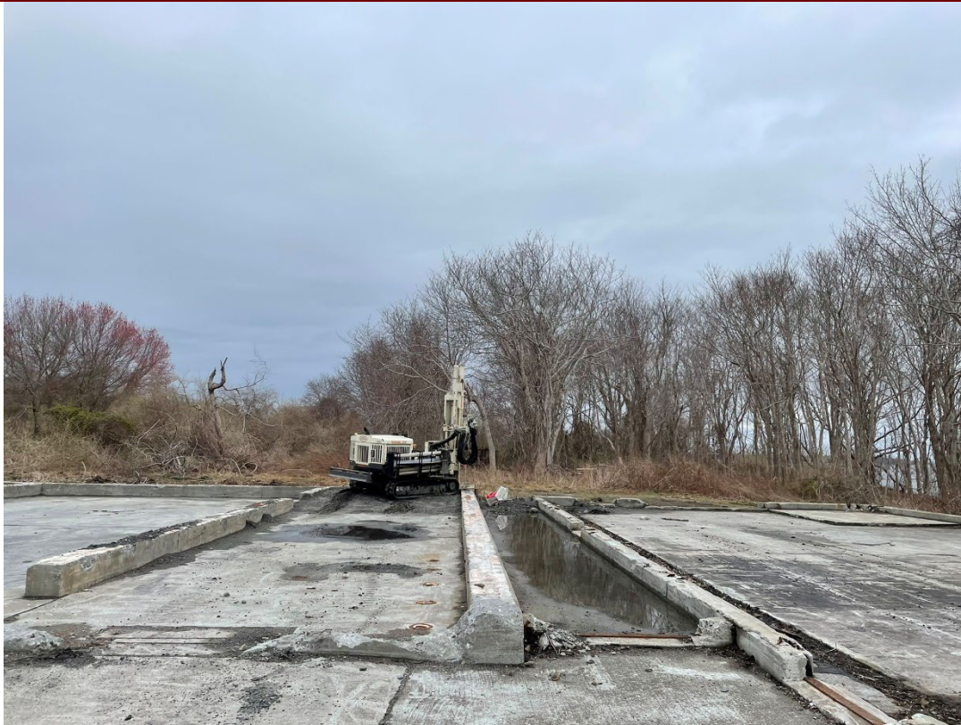
9. View of boring advancement at Fire Station (NED 12)
