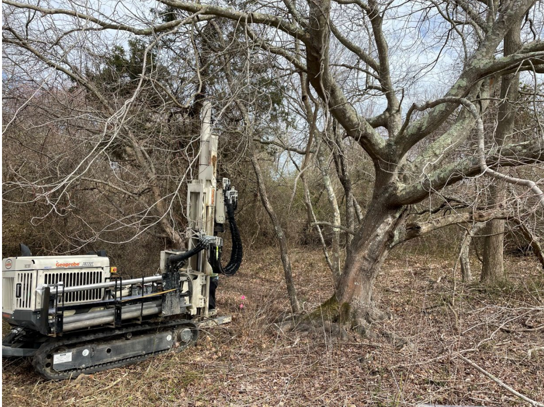
7. View of boring advancement at Coal Storage North (NED 1)
