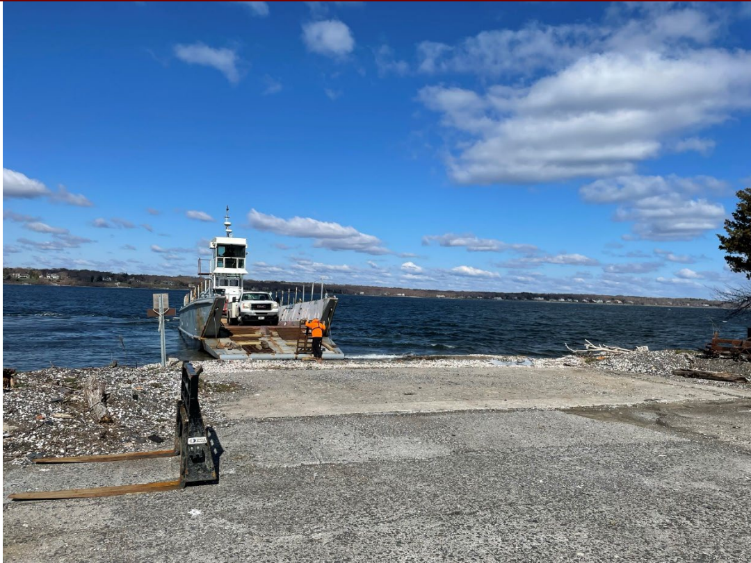
3. View of drilling equipment delivered to the island on April 4, 2022
