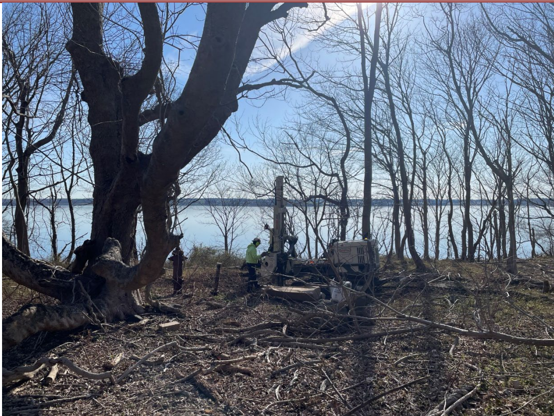
6. View of boring advancement at former Quonset Huts (NED 11)
