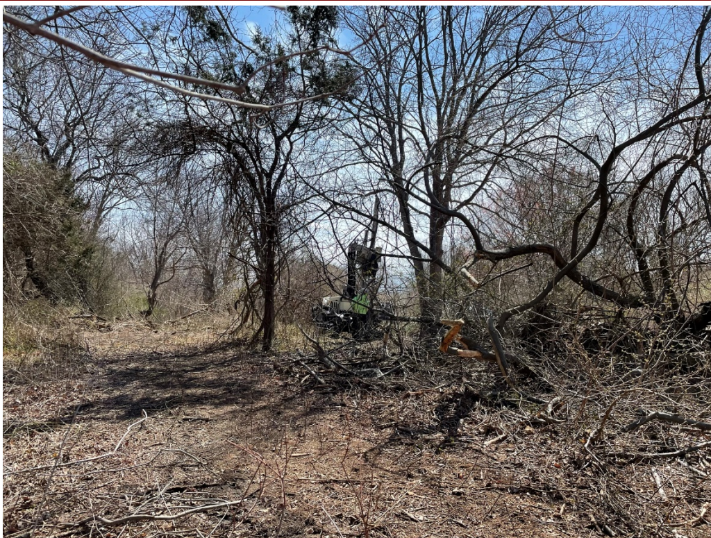
4. View of boring advancement at NED 01
