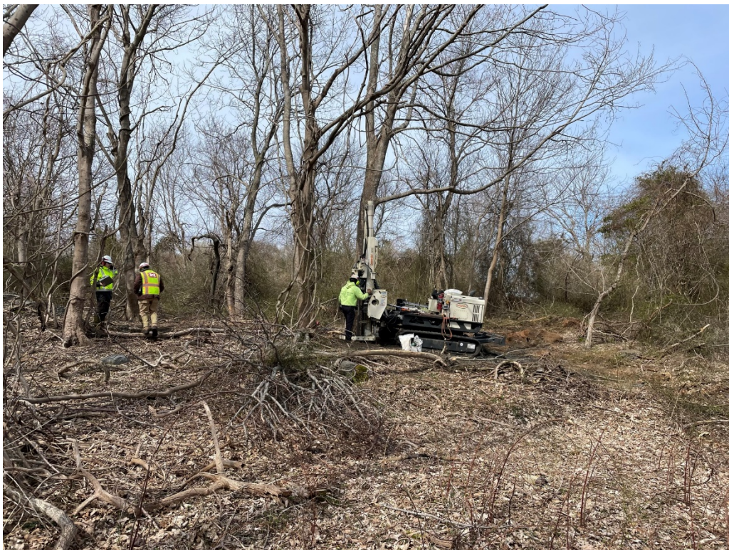
3. View of boring advancement at 11SB2
