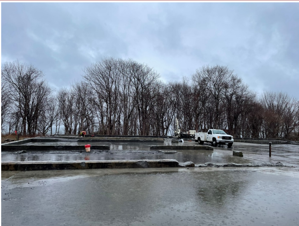
4. View of concrete coring activities at NED 12
